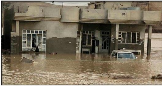
Picture 1. Shows houses flooded
